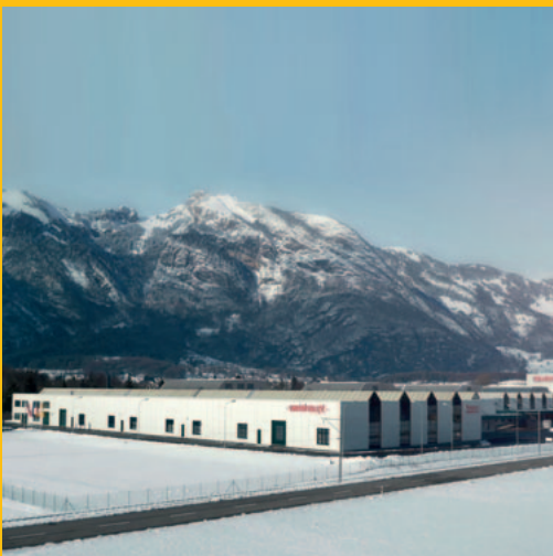
Weishaupt has manufacturing facilities in Germany and Switzerland
