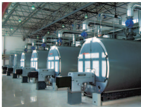
Xi'an, central China: The seven WKG gas burners in this heating centre provide more than 50 000 residents in the Zi Wei garden district with 115 MW of heat
