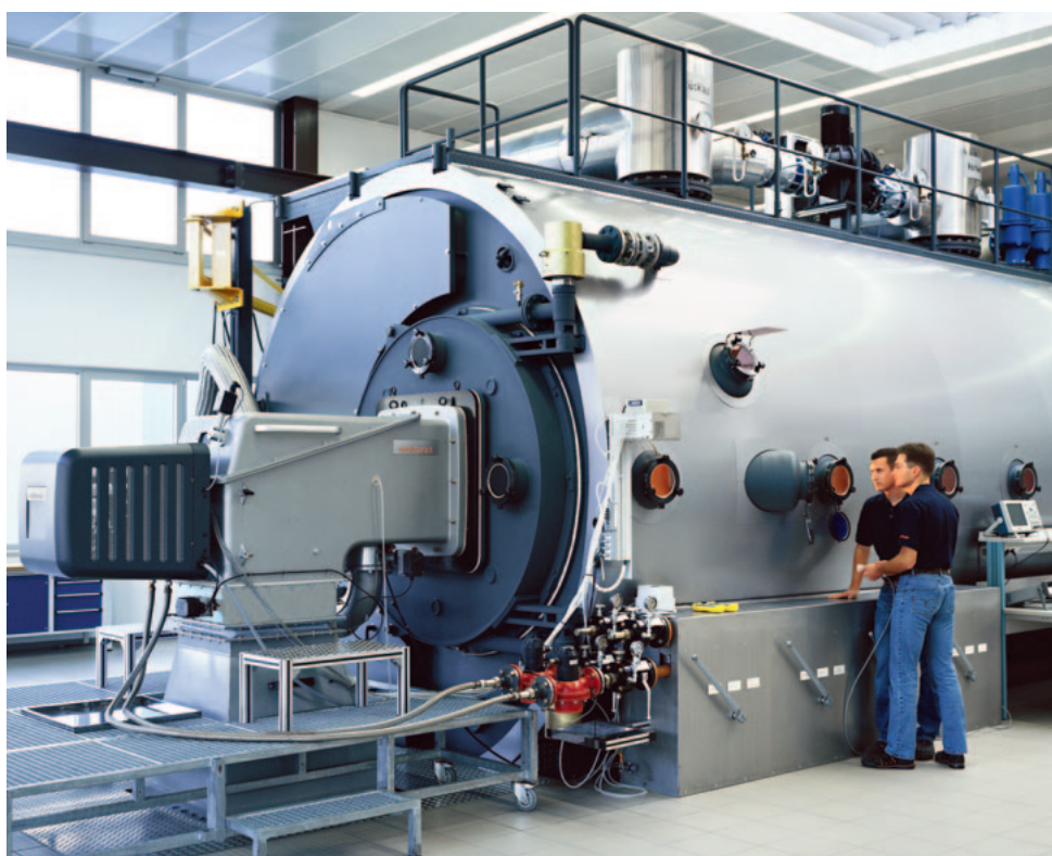
Xi'an, central China: The seven WKG gas burners in this heating centre provide more than 50 000 residents in the Zi Wei garden district with 115 MW of heat
